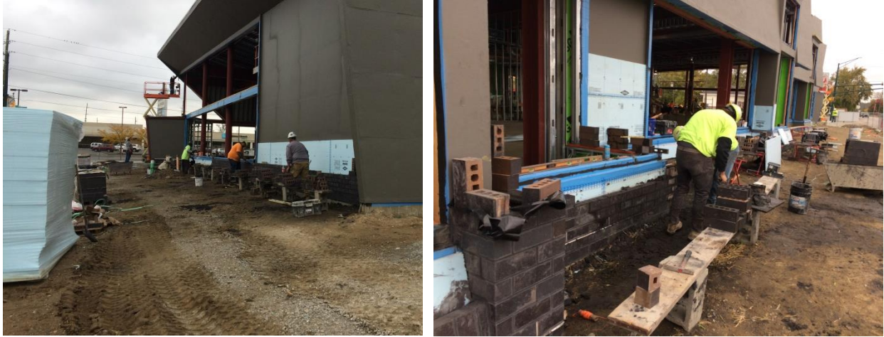
Project Site on October 29, 2019 View of the Masons Working on the North and East Elevations.
