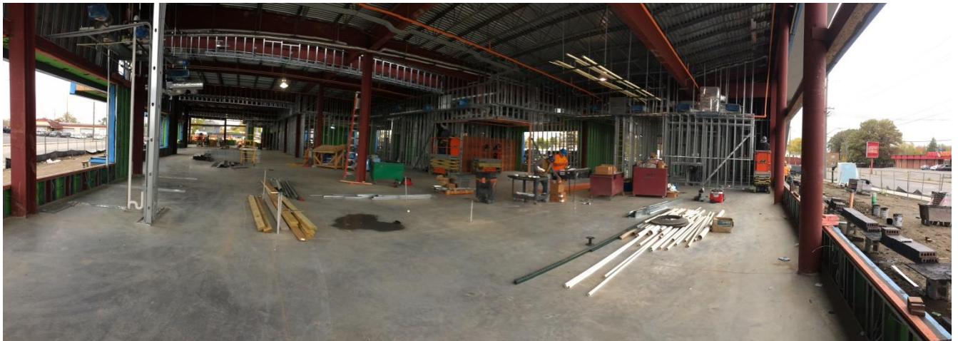
Project Site on October 29, 2019 Interior Panoramic View from the Sherman Entrance.
